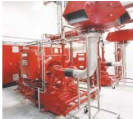
700 HP (520 kW) Turbo Air® Compressors installed at plastics processing facility.
